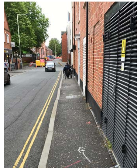
6 - Cross gradient 1:6 on footpath
