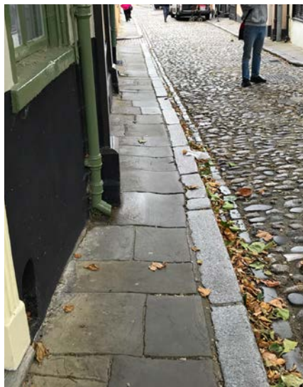
2 - Cobble stones. Pavement width restriction 600mm (alternate route via The Monastery shown in orange)
